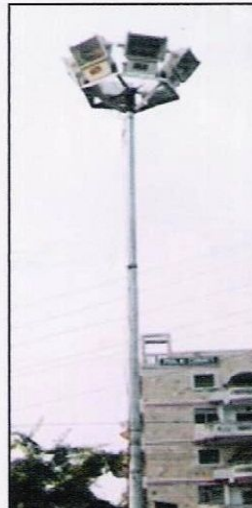
SEMI HIGH-MAST height : 8-12 mtr
